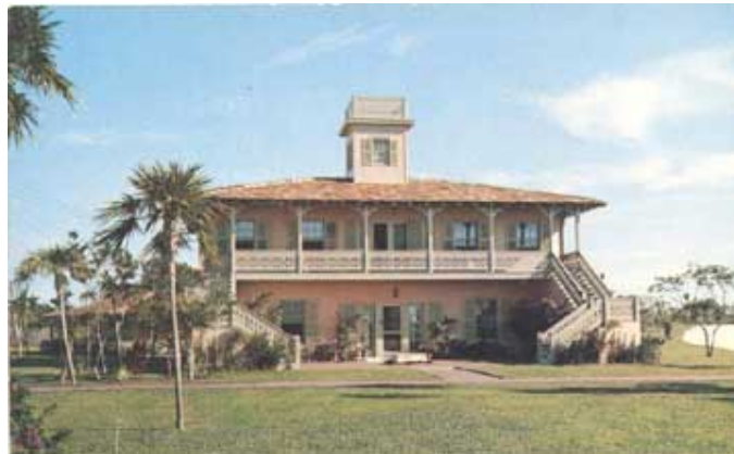
DUCK KEY ADMINISTRATION BUILDING An excellent example of West Indies architecture that predominates on this tropical island 90 miles South of Miami at Tom's Harbor in the Florida Keys. The Administration Building is two stories high with "Captain's Walk" and has an entrance courtyard symbolic of Caribbean island architecture. Floor tiles for its main lobby were imported from Cuba as was most of the French Provincial and Spanish furniture and decorations. There are twin offices in the building, twin apartments with overhanging porches and a beautiful entrance lobby. Duck Key is a residential, motel, apartment and business center development complete with yacht harbor and 9-hole golf course.
